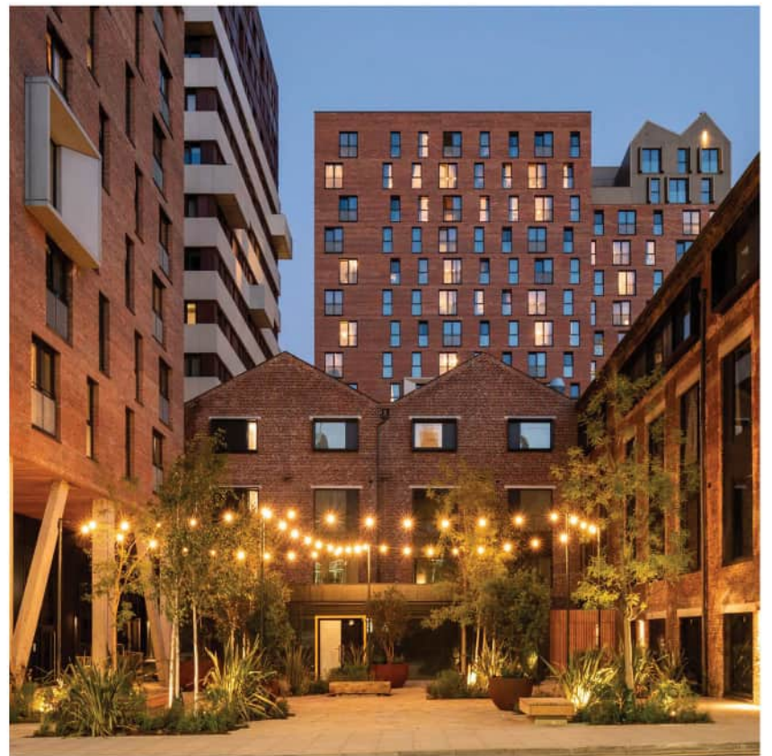
KAMPUS Apartments, Manchester Mecanool | © Greg Holmes Photography
